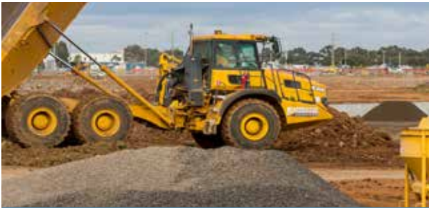
Cement & Concrete / Construction
